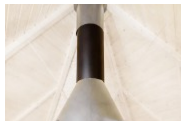
Grill Chimney Extension
